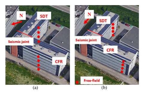
Figure 4 – View on the building, SDT and CFR sides, seismic joint position, position and direction of measurements for ambient vibration tests at each floor before and after the May 20 earthquake (a), and after the damage repair(b).
