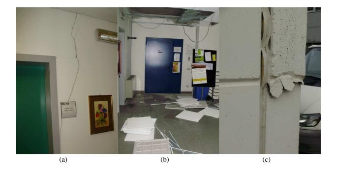
Figure 3 – Damage occurred on the SDT side of the investigated building. (a) curtain wall of the chemistry laboratory at the ground floor; (b) SDT side entrance at the second floor; (c) detail of one of the external wall.
